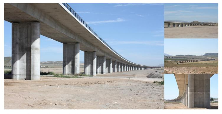
The section Villena-Sax of the High Speed Railway Line Madrid - Levante includes the construction of two great length viaducts: Acequia del Rey and Cordel de Sax. The first one has a total length of 1,394m divided into 44 spans with the following arrangement: 25m+42x32m+25m. The Viaduct over the Cordel del Sax has a total length of 1,458m divided into 46 sections with the corresponding span lengths: 25m+44x32m+25m.
